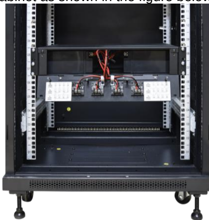
Fig. 3. The battery mounting method.
